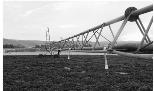
Figure 4 - PVC pipe leading water under the pivot, a local DIY adjustment to avoid corrosion caused by saline irrigation water.
