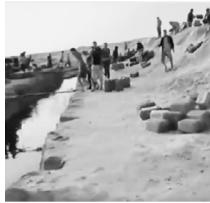
Figure 3 - Fuel smugglers at “Dhahret El Khos” (through the protective wall).
